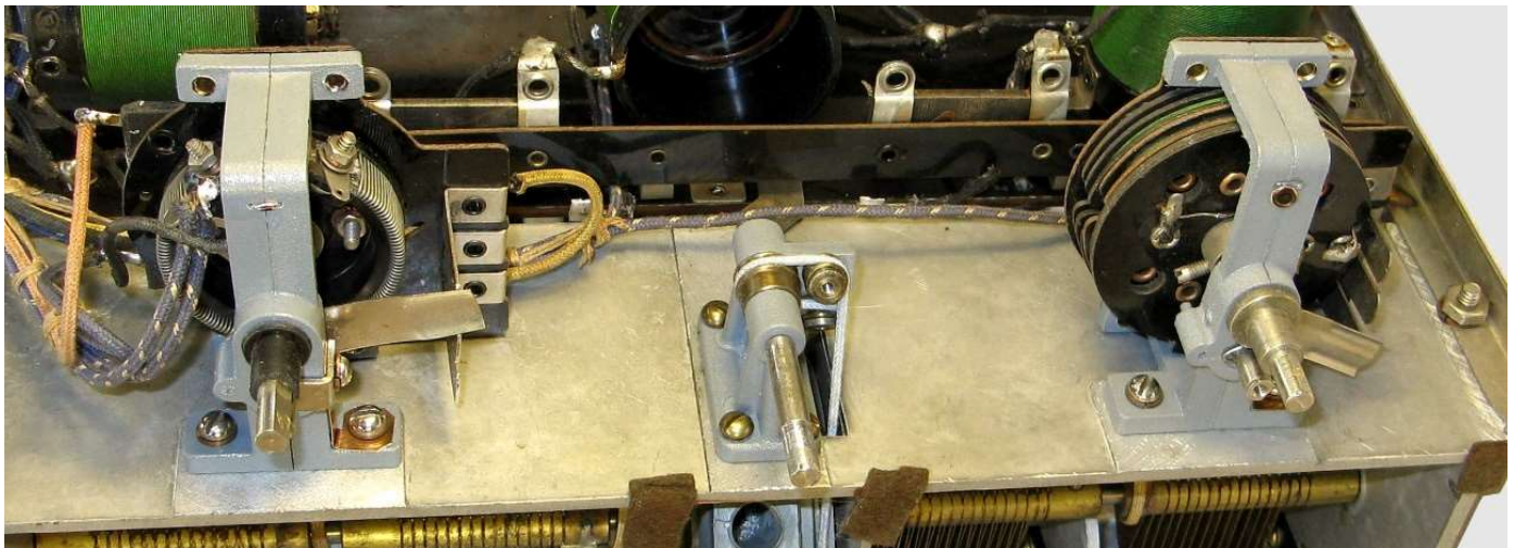
Figure 5 - 3D Printed Parts installed. Left, rheostat bracket - Center, Drum drive, Right, Variometer bracket.
