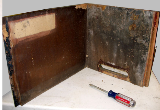
Rotted veneer ply.
